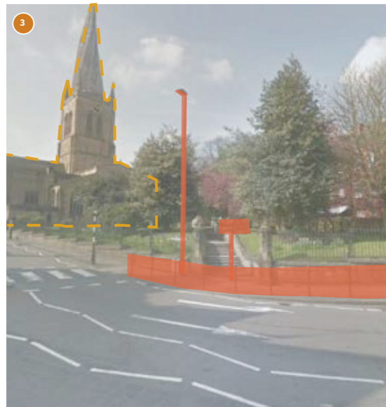
ROADSIDE RAILINGS, LIGHTING AND POORLY PLACED SIGNAGE HIDES THE CHURCH ENTRANCE AND VIEWS OF THE MEMORIAL
