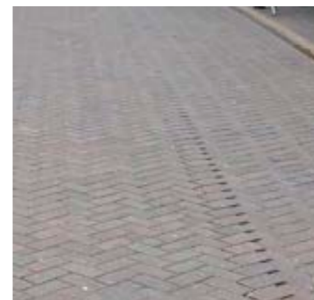
HERRINGBONE CONCRETE PAVERS ON BURLINGTON STREET
