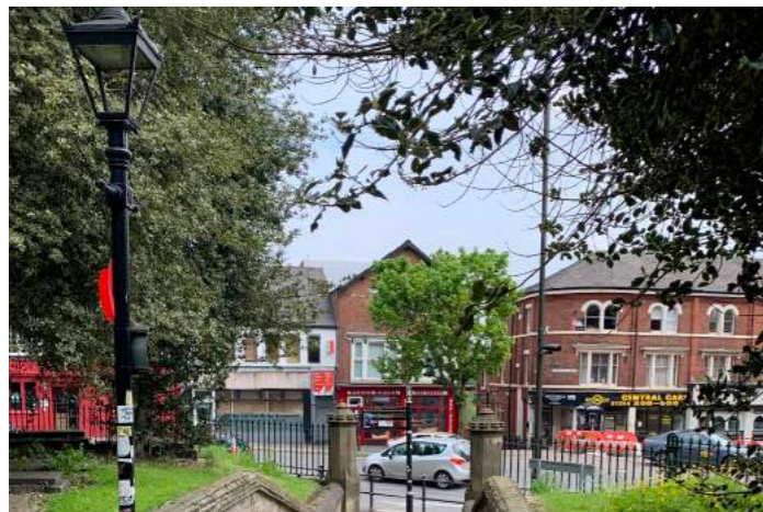
FOOTPATH LIGHTING INFRASTRUCTURE IN ALL SAINT'S & ST. MARY'S
