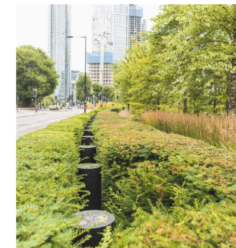
Bollards concealed in hedging
