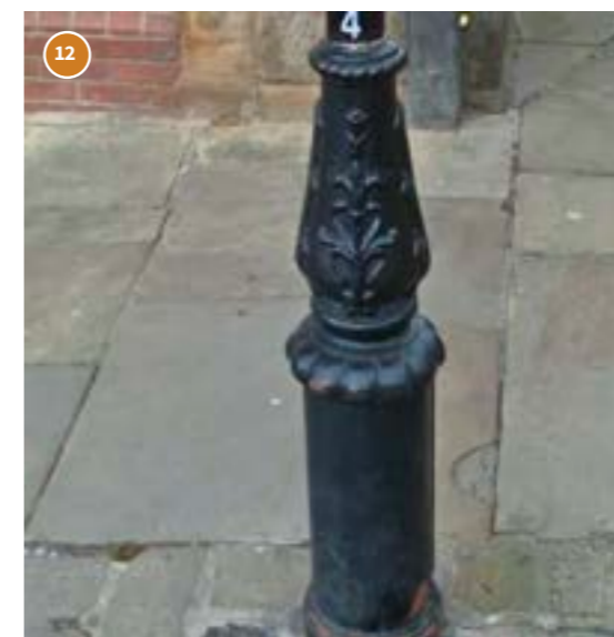
12 TRADITIONAL DETAILING TO BASE OF SOME COLUMNS
