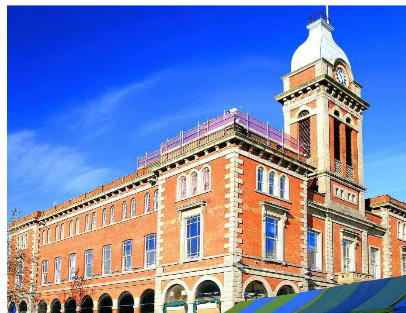
Chesterfield Market Hall's historic facade
