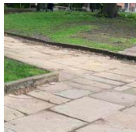
CIRCULATION YORKSTONE SLABS AT ST MARY AND ALL SAINTS CHURCH
