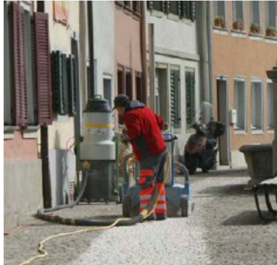
SETTS BEING GROUND IN-SITU IN A GERMAN TOWN; OPTION ONE
