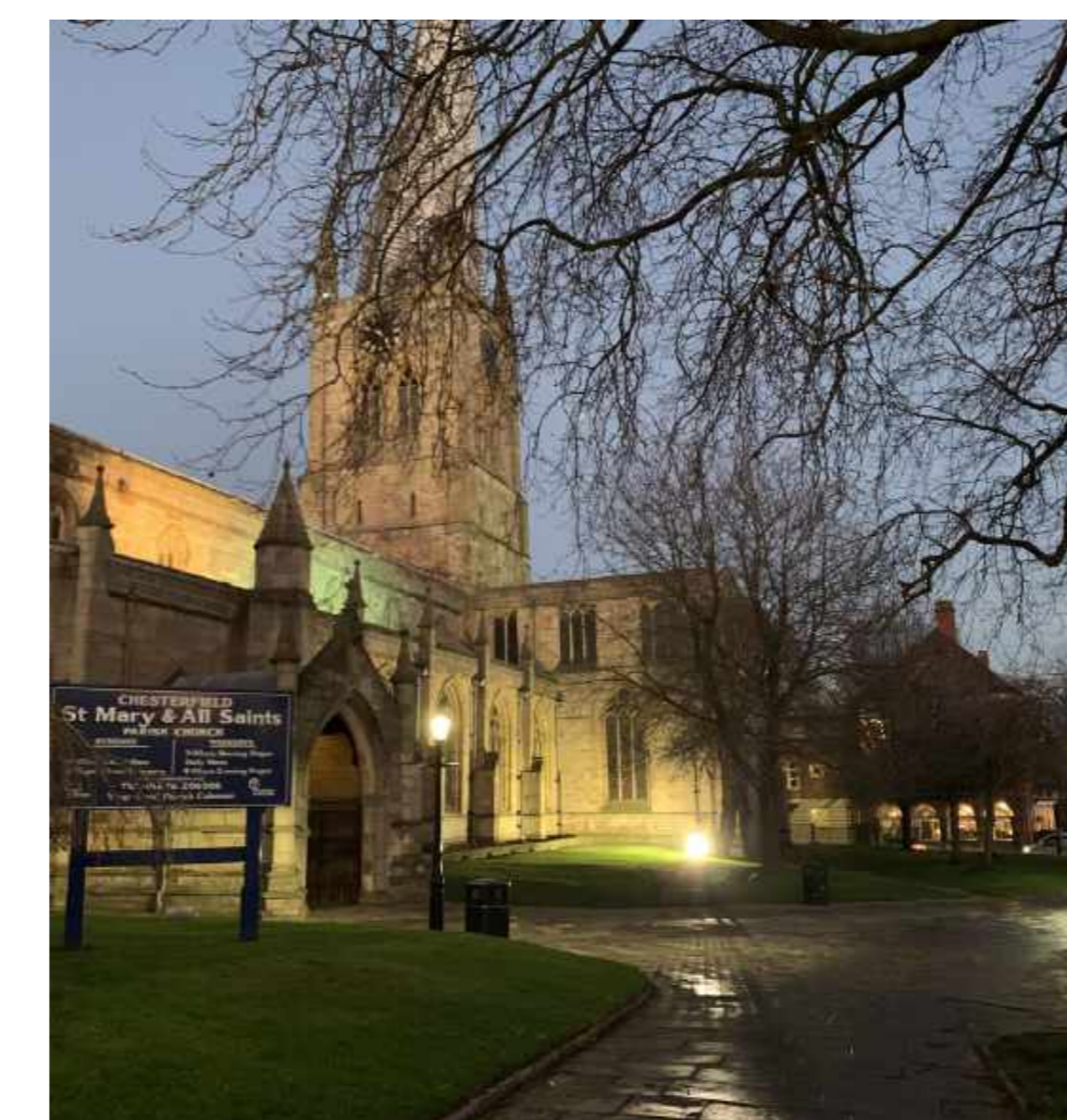
Existing Church architectural lighting adds interest but could be improved
