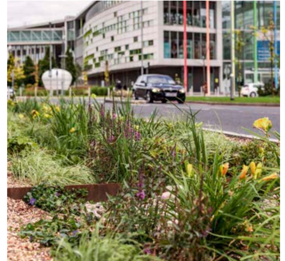
RAINGARDENS ADJACENT TO ROADS TO CATCH ANF FILTER RUN-OFF
