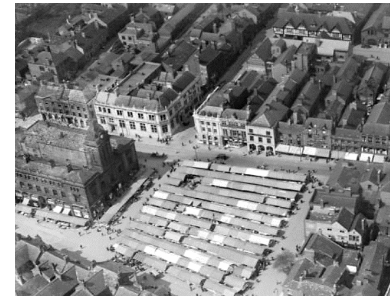
1928 Market aerial view
