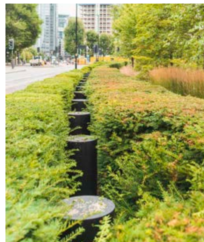
BOLLARDS CONCEALED IN HEDGING
